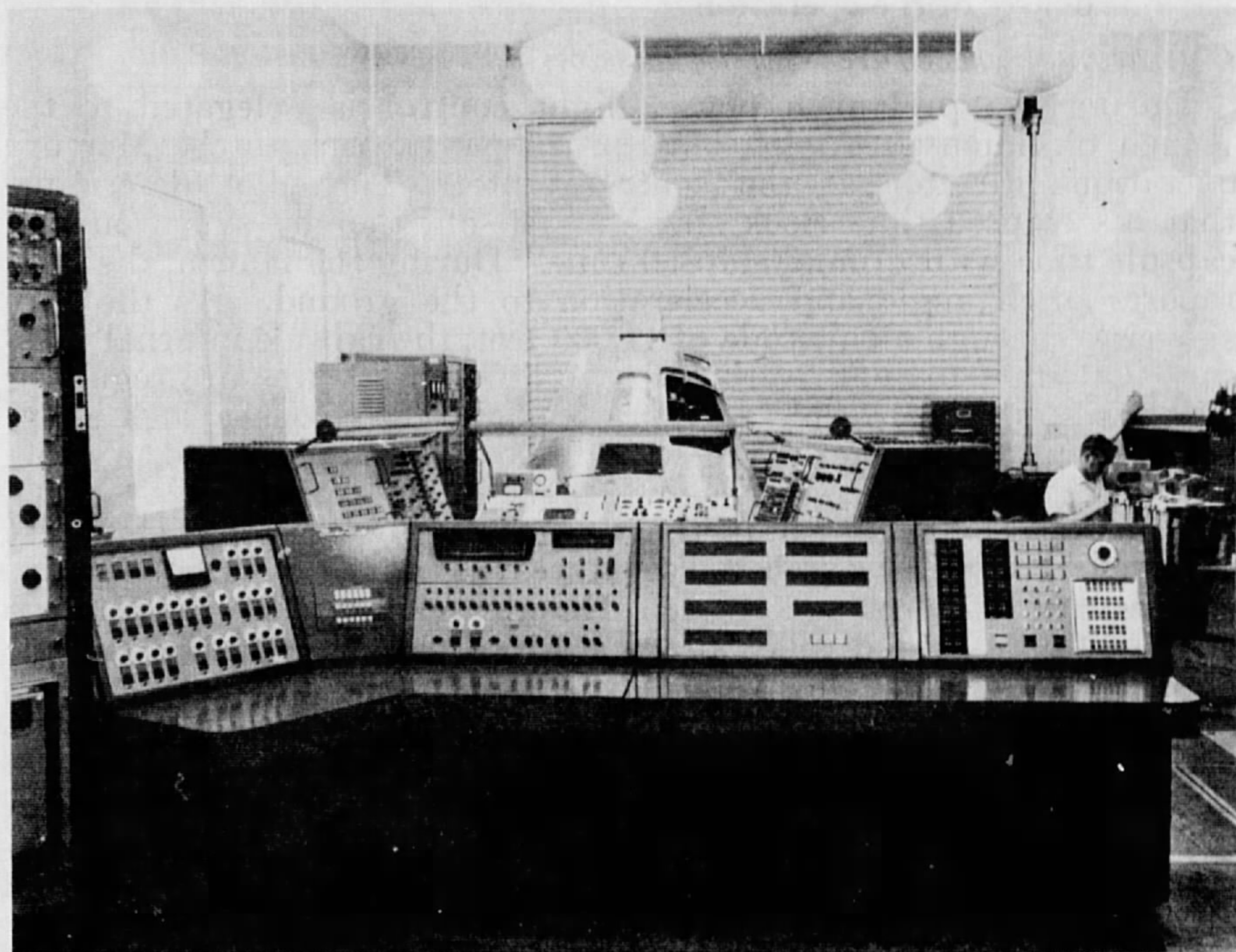
FIGURE 25.—Procedures trainer console installation.
