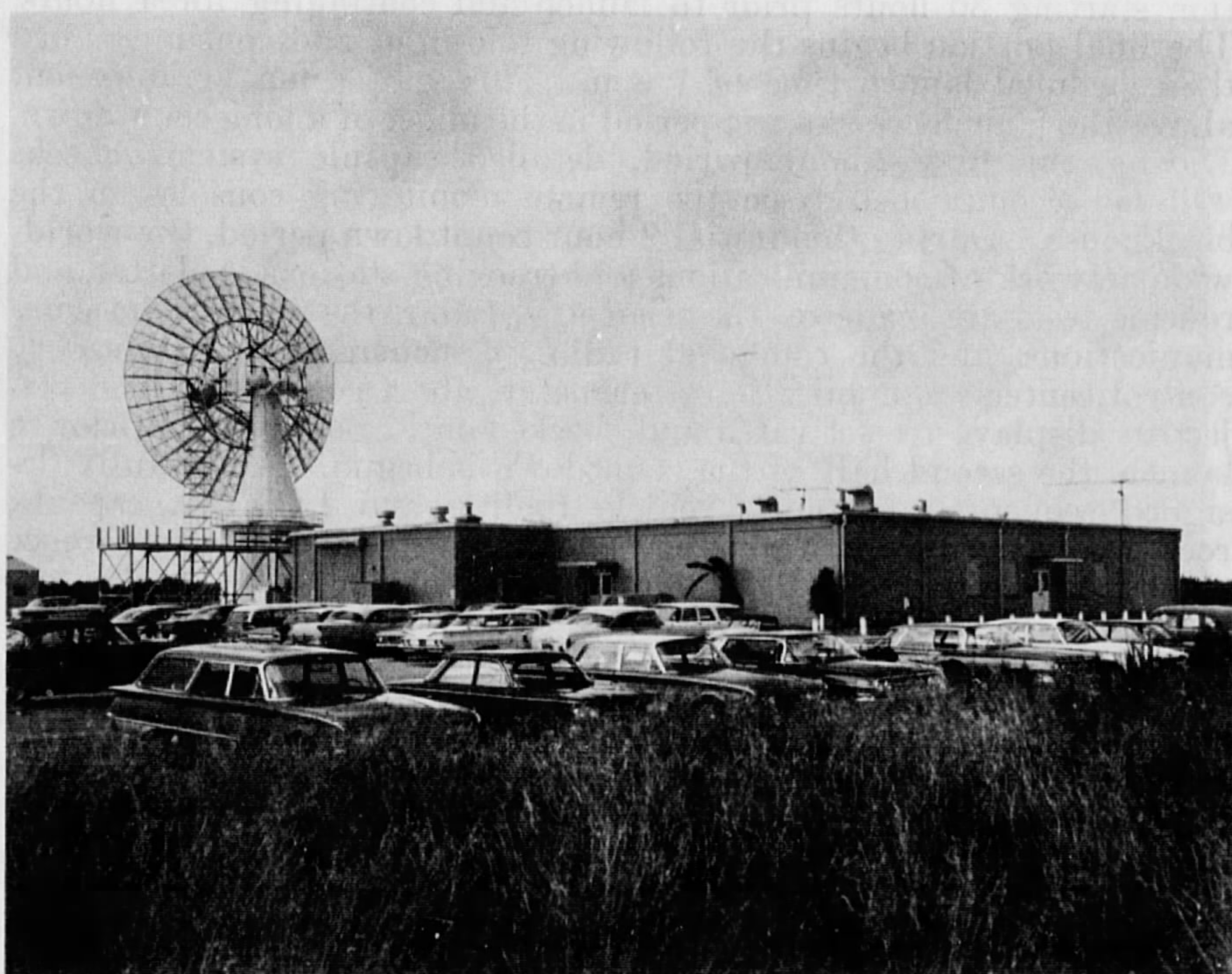
FIGURE 21.—Mercury control center at Cape Canaveral.
