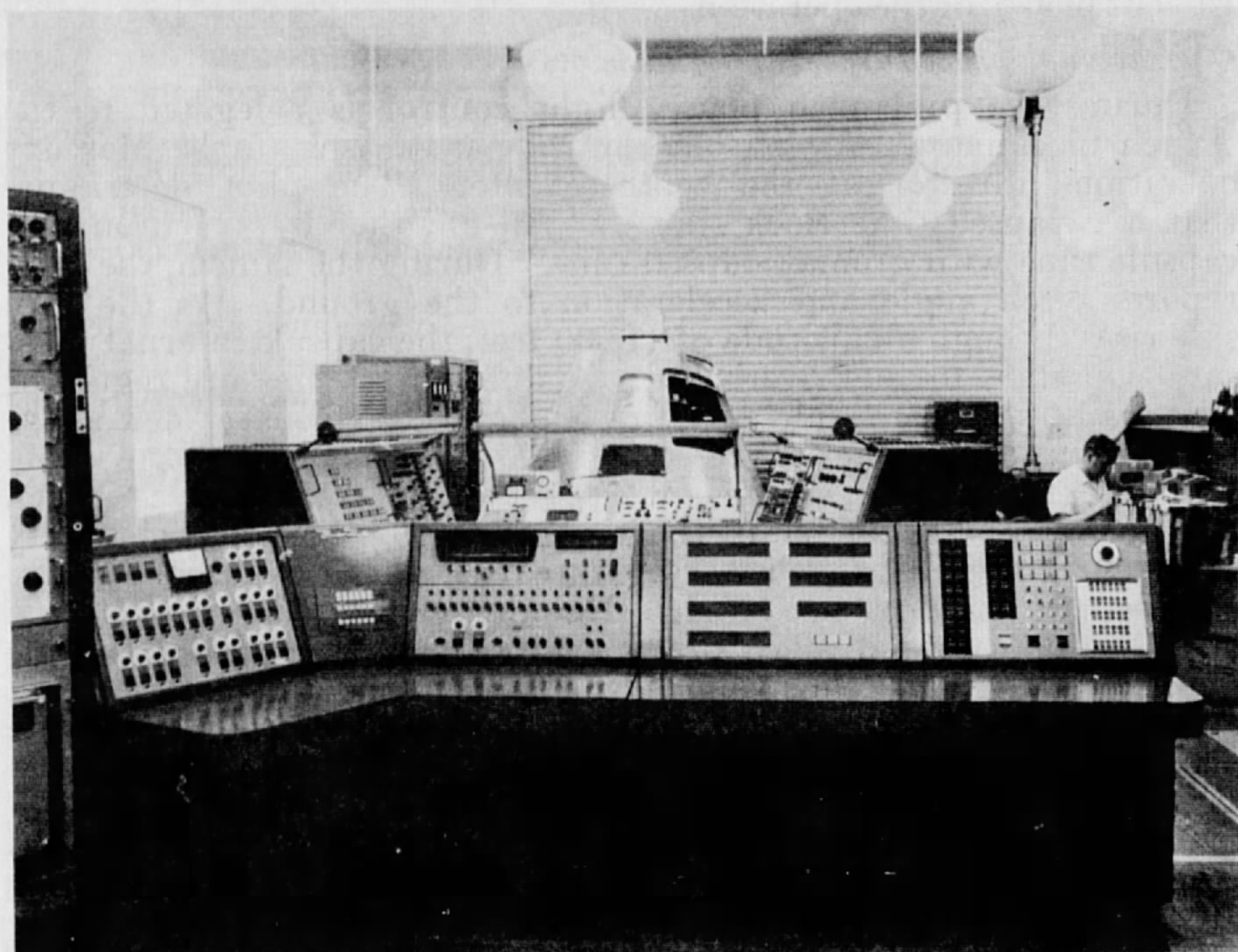
FIGURE 25.—Procedures trainer console installation.
