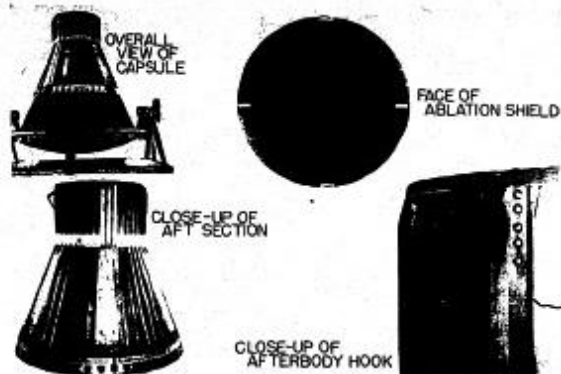
FIGURE 4.—Detailed photographs of recovered Big Joe capsule.
